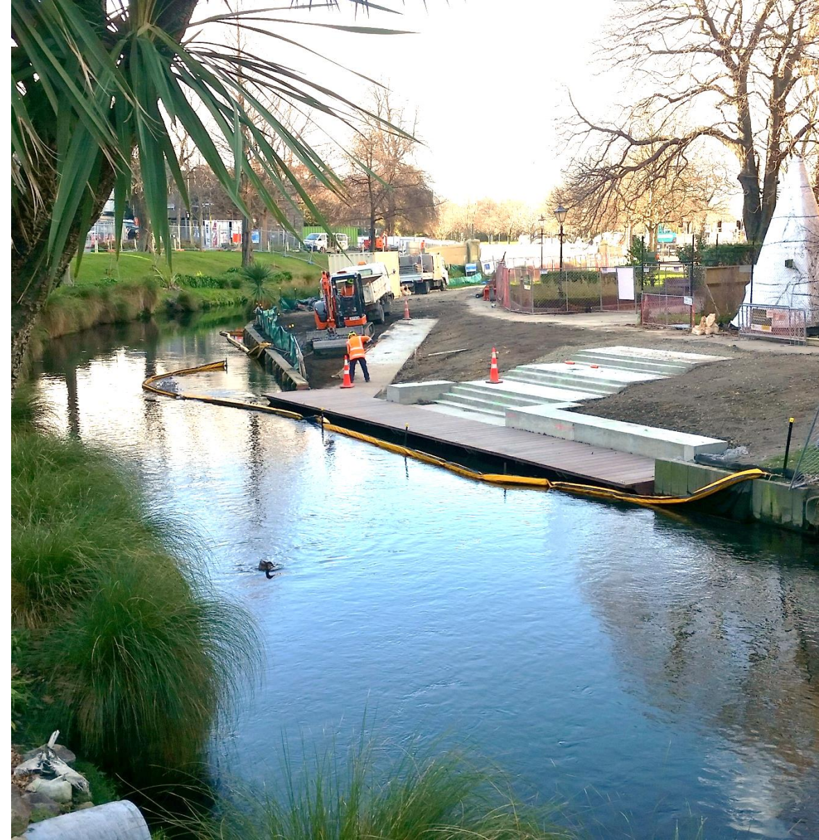
TTT Poles used in a Deep Pile Foundation – Commercial Site, Avon River, Christchurch New Zealand H6 TTT MultiPole Uglies 4.8m long x 250mm diameter were used for a punt stop and river wall.
