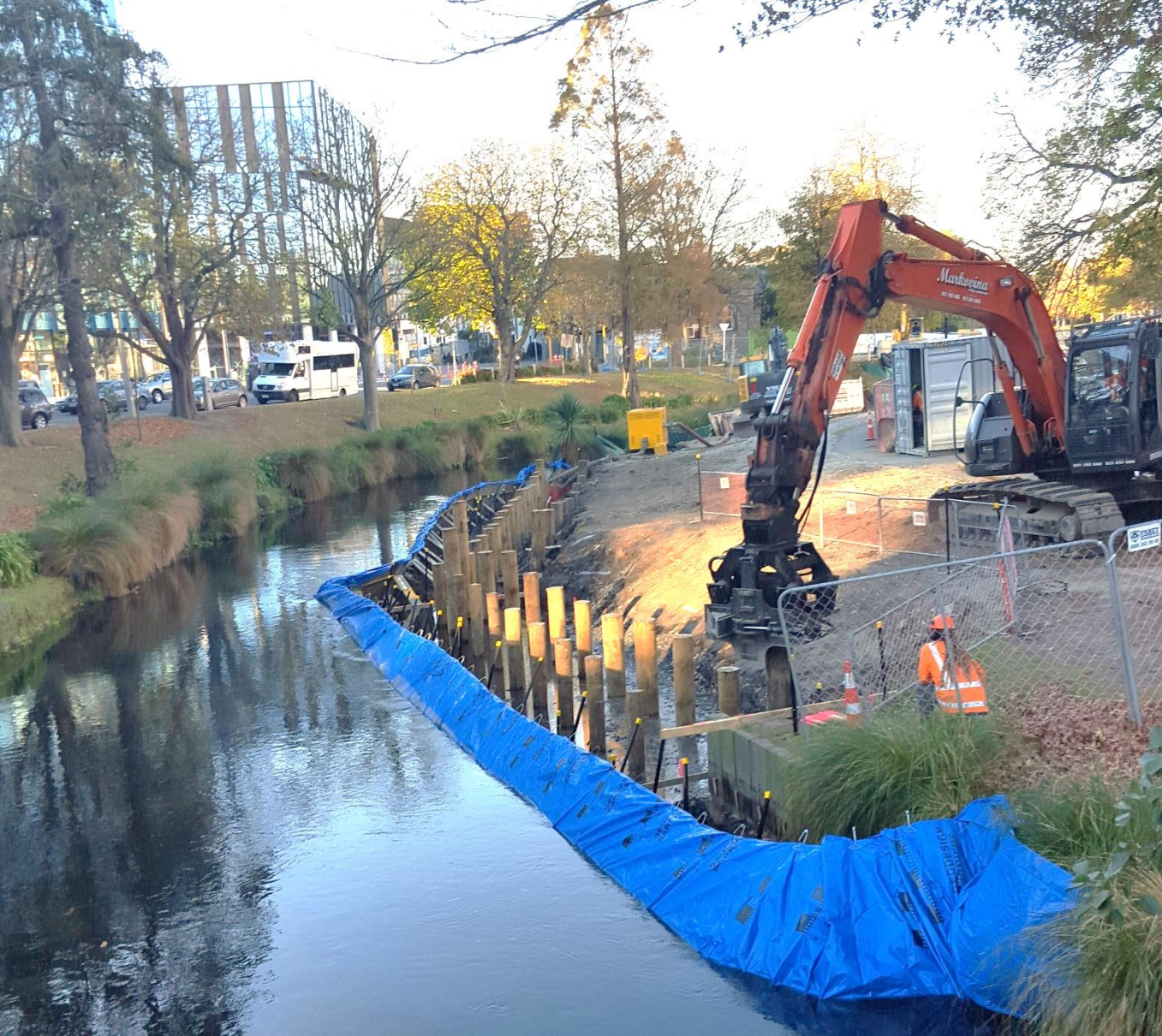
TTT Poles used in a Deep Pile Foundation – Commercial Site, Avon River, Christchurch New Zealand H6 TTT MultiPole Uglies 4.8m long x 250mm diameter were used for a punt stop and river wall.
